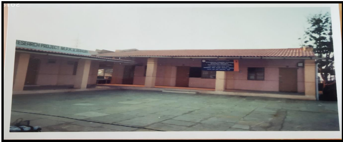
Photo: Project Old building
